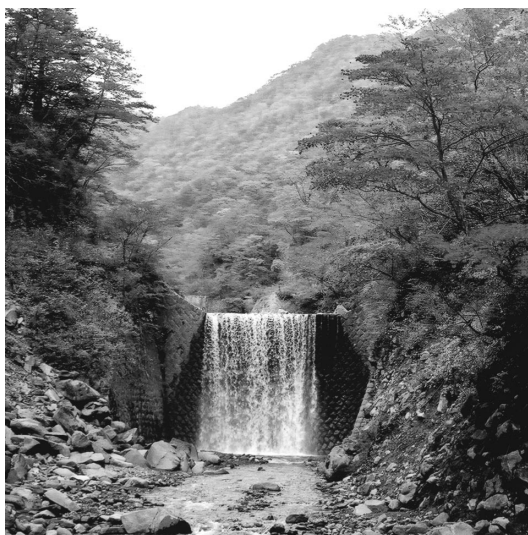
釜ツ沢下流砂防堰堤
